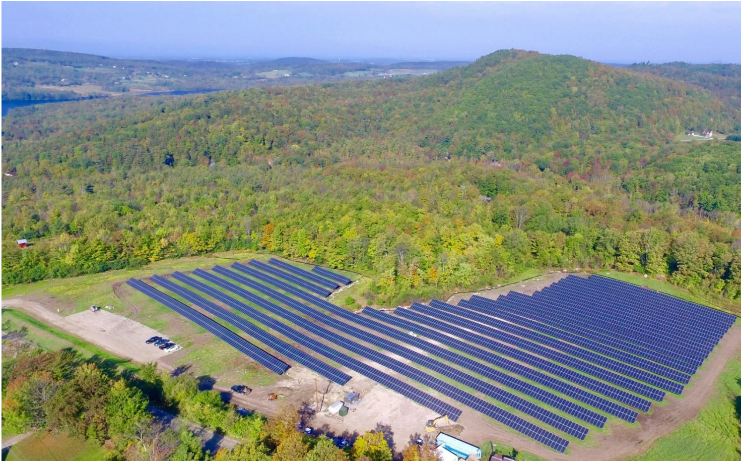
Photo: Courtesy of Encore Renewable Energy
